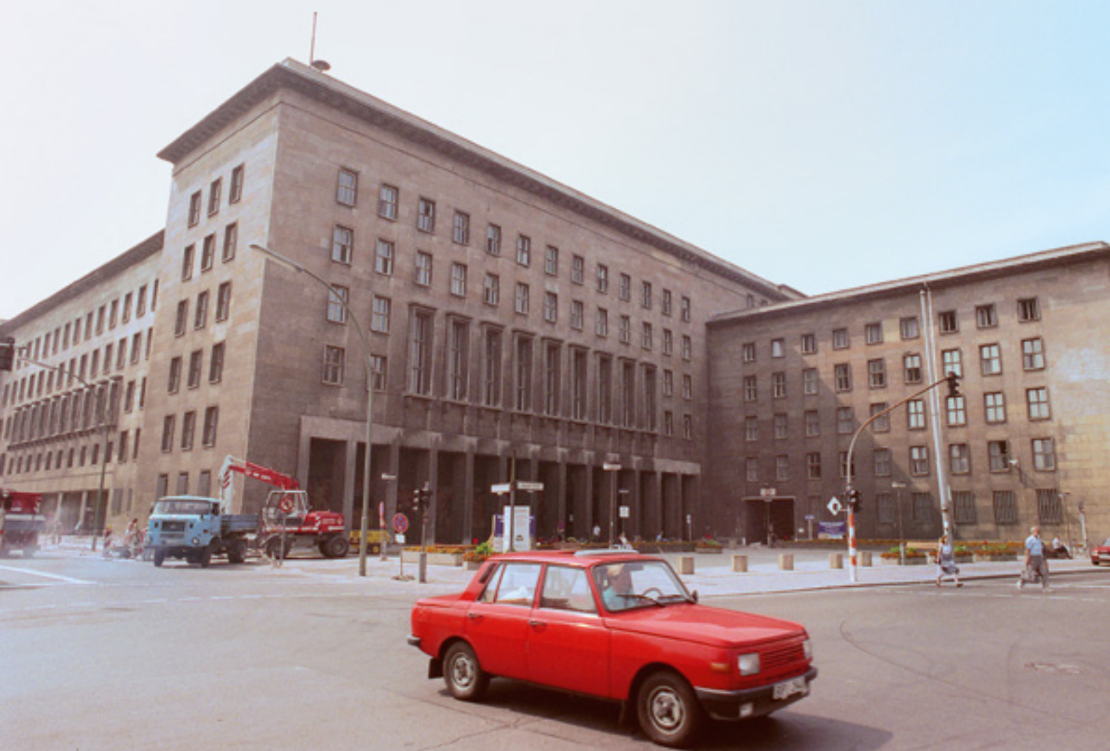
View of the former House of Ministries at the intersection of Leipziger Strasse and Wilhelmstrasse in August 1991.
