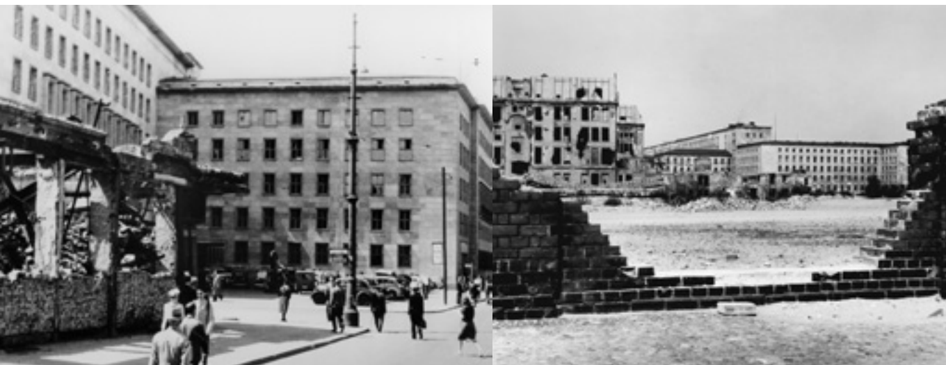
Damage done to the former Reich Aviation Ministry.
